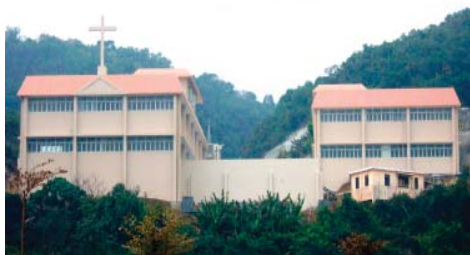
Building of the male center
