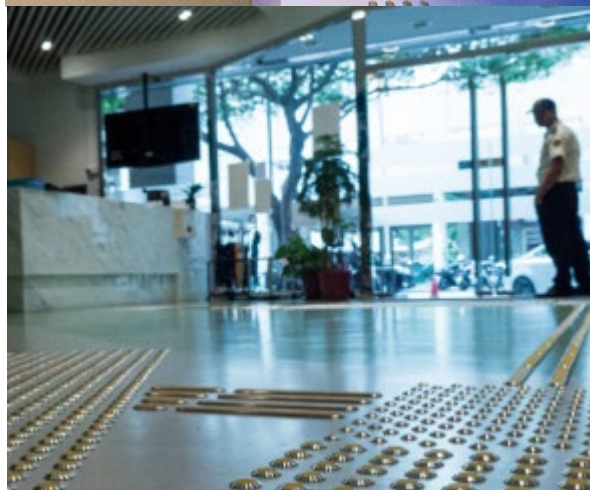
Provision of tactile warning strip
